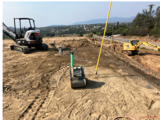
Rawlings Backfill at SDG&E Pole
