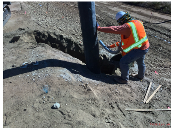
Installation of Underground Electrical Utilities
