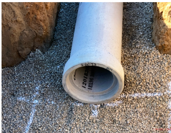
Storm Drain Piping
