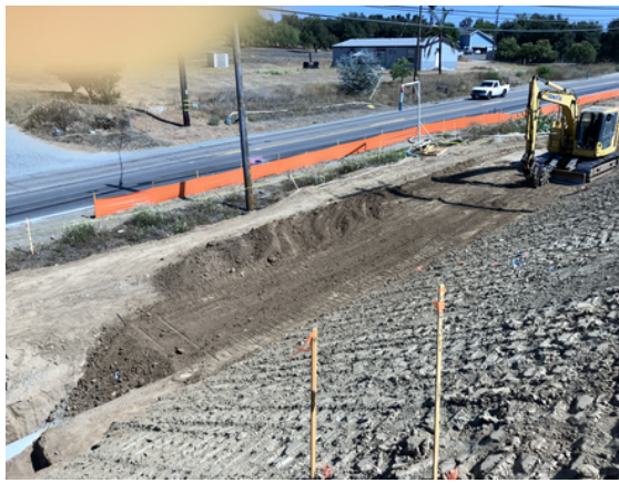
Storm Drain Backfill
